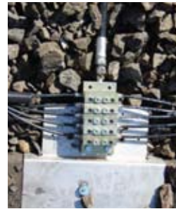
Lincoln UV Modular Progressive Divider Valve
