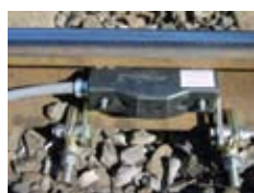
01-086001 Axle Counter for TOR Lubrication System
