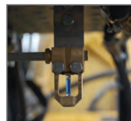
Heat capsule detector installation
