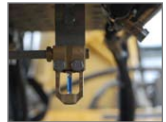
Heat capsule detector installation
